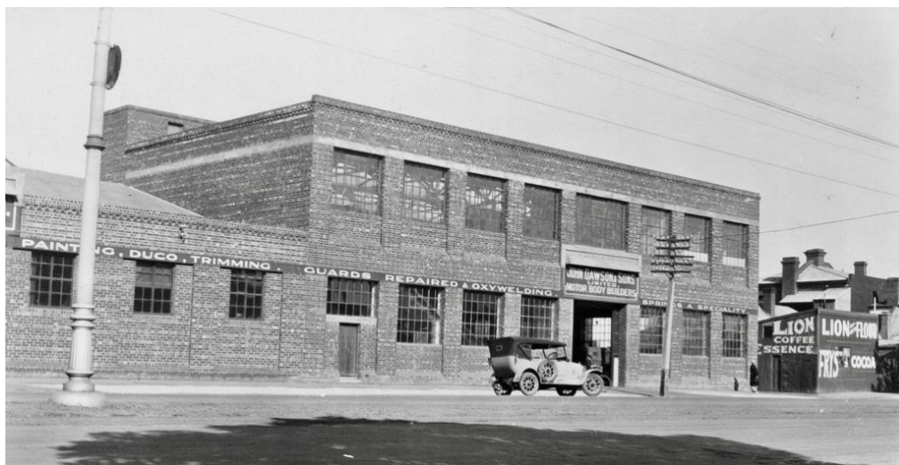
Below: The premises of John Dawson & Sons, Limited, Motor Body Builders, Wakefield Street, Adelaide, in about 1927. The firm began business in 1900. [State Library of South Australia.]
