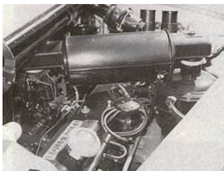
4BP3: the straight-eight engine. Note the oil-bath air cleaner, fitted for dusty countries. Silver Wraith and Silver Dawn owners will notice similarities.
